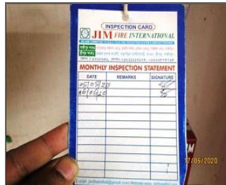
Photo of the inside of the main production hall Fire Equipment Inspection record.JPG
