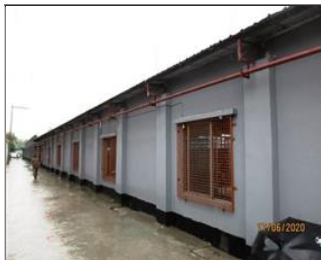
External photo(s) of the production unit(s) Factory Main production shed.JPG
