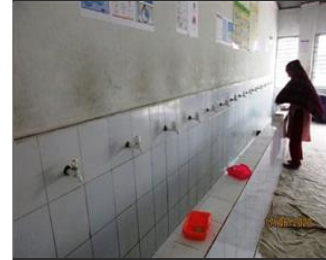
Photo of the canteen (if applicable) Wash facility at workers dining.JPG
