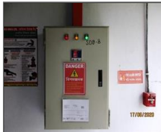
Photo of the inside of the main production hall Danger Sign.JPG
